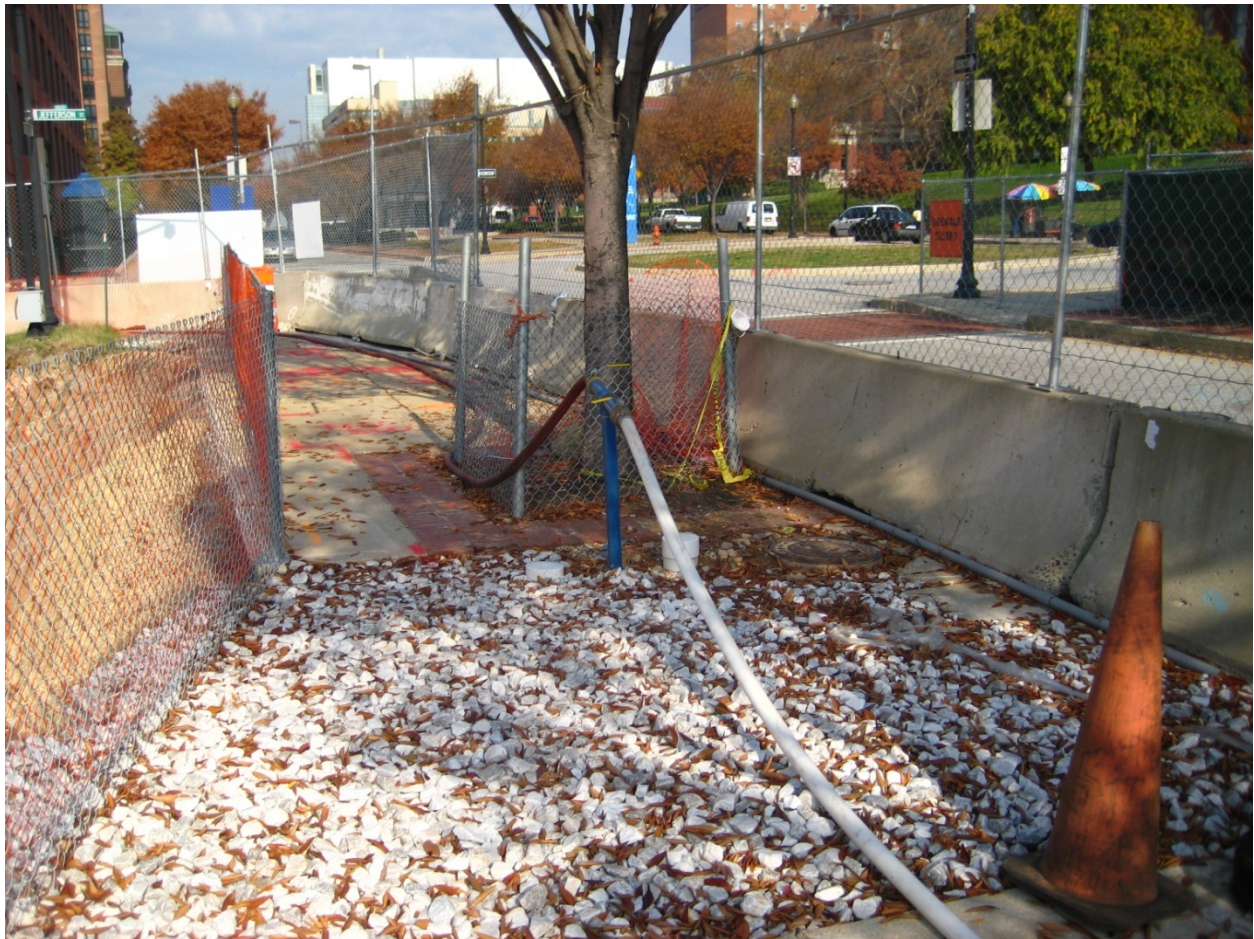
Temporary Water Connection
