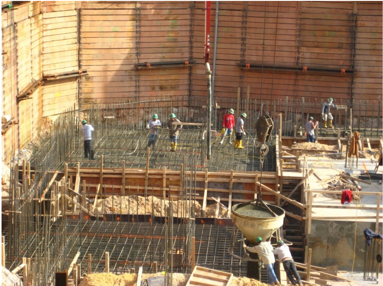
Workers place concrete for mat foundations
