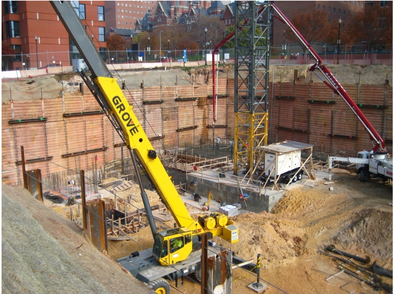
Looking Northeast from center of site
