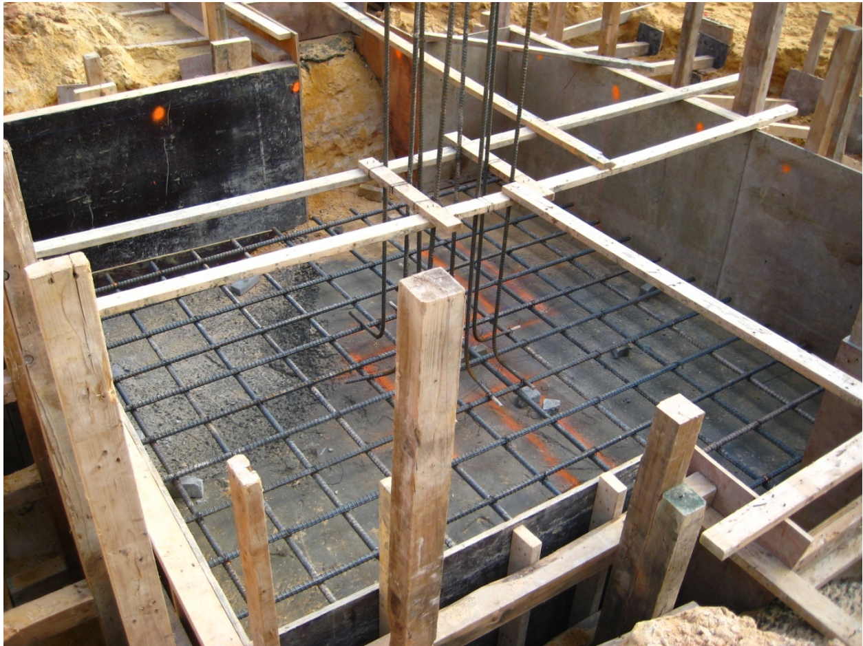
Mud mat under mat footing form
